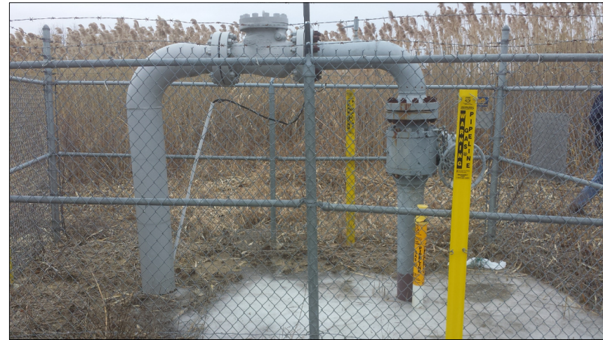
TAP STATION – EXISTING CONDITIONS
