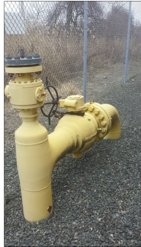
VALVE STATION – EXISTING CONDITIONS
