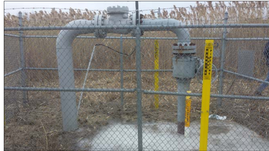
TAP STATION – EXISTING CONDITIONS
