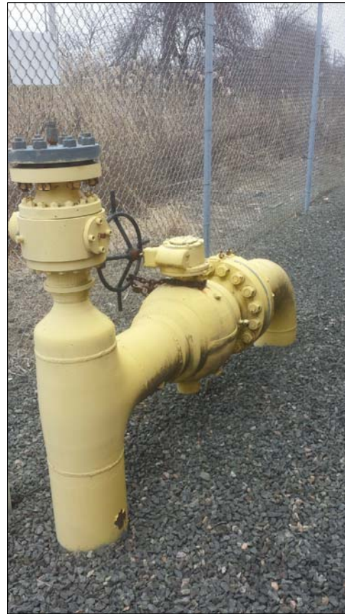
VALVE STATION – EXISTING CONDITIONS
